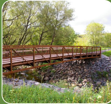
Example of the pedestrian bridge.
